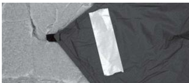
Repair Tear in Tarp
