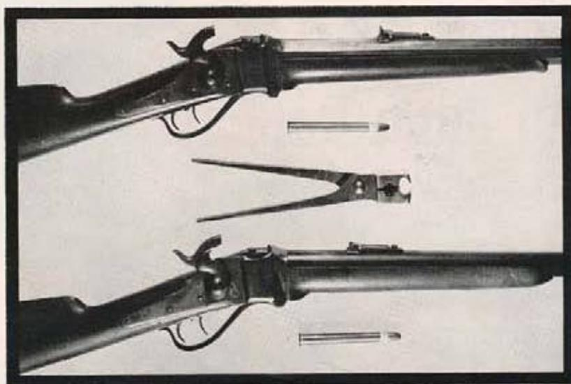
Octagon barrel (top) was preferred on Sharps over less expensive round barrel. Bullets were made on the range, using mould shown.
